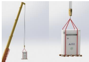
Lifting by crane
